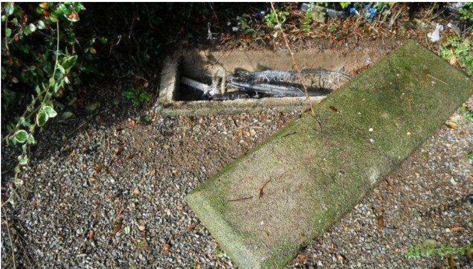
Photograph 2: Wellhead with concrete slab cover and potential entry of surface water to well
