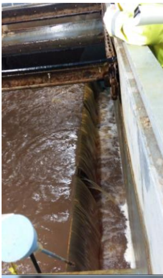
Photo 3 Backwash on DAFF Unit No 1 – water escapes via gap in weir
